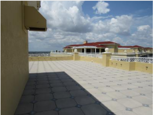
Private Roof Terrace - Pedestal paver roof system (mod. bit. below pedestal pavers).
