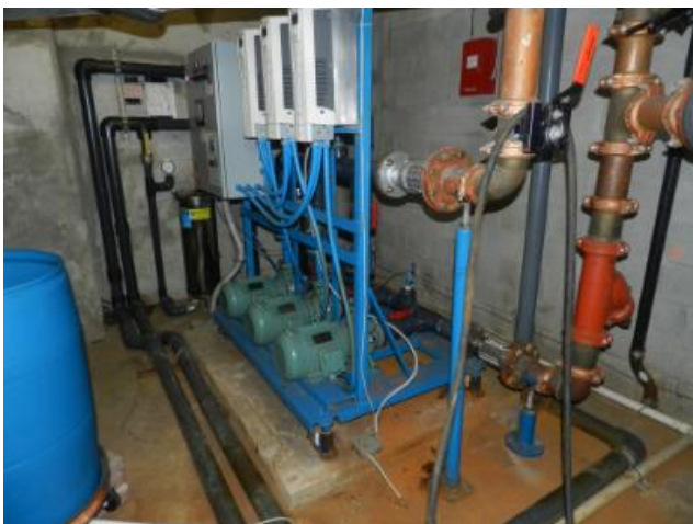
Typical variable speed domestic water pump system.
