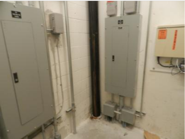
Typical sanitary plumbing line and corrosion or unknown staining on the exterior.
