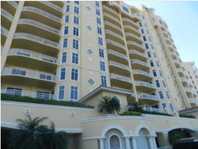
Typical exterior glass block openings.
