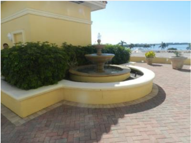
Elevated planters above parking garage. Staining and cracked planter wall cap.
