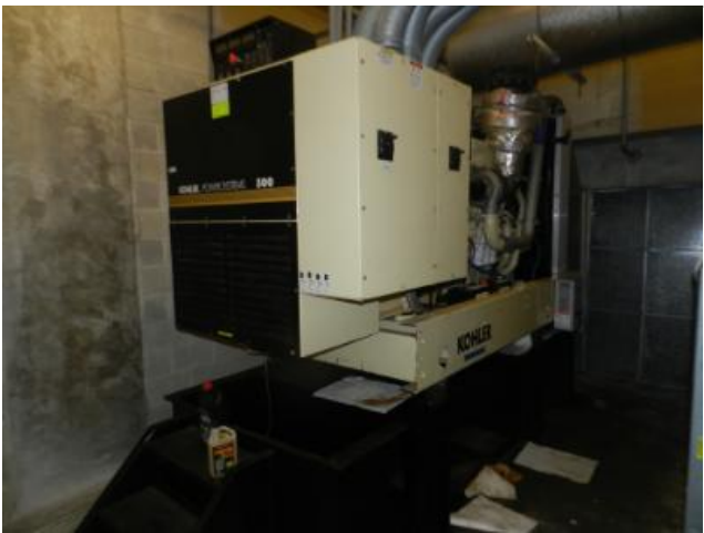
Typical emergency diesel generator.
