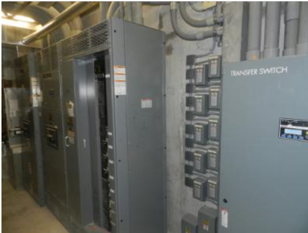
Main electrical disconnects, main distribution panel, and transfer switch.
