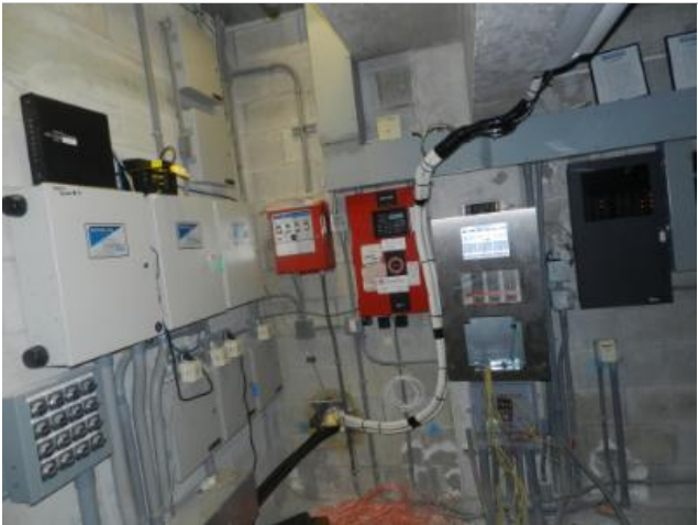
Typical Fire Alarm Control Panel.
