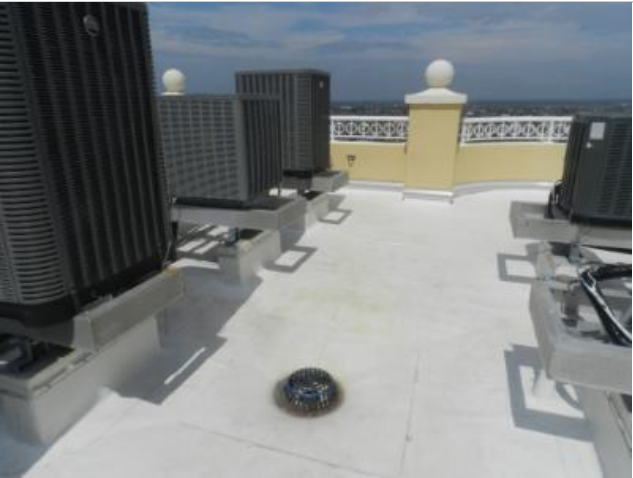
Typical TPO roof covering system and HVAC stands.
