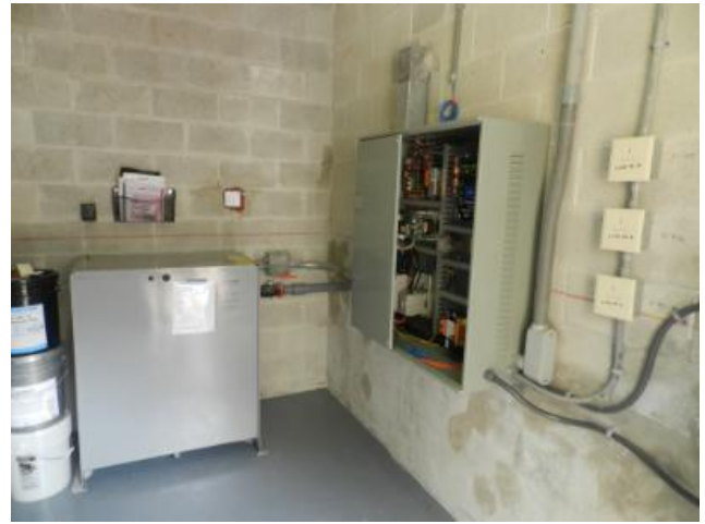
Hydraulic elevator controls and pump housing container.
