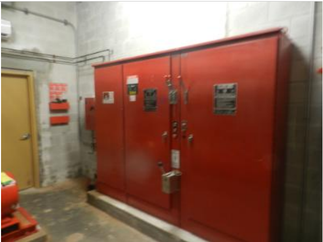
Fire pump main controls.
