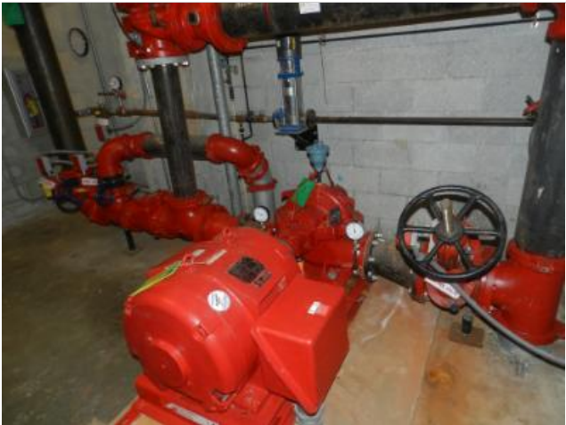
Typical emergency fire pump.
