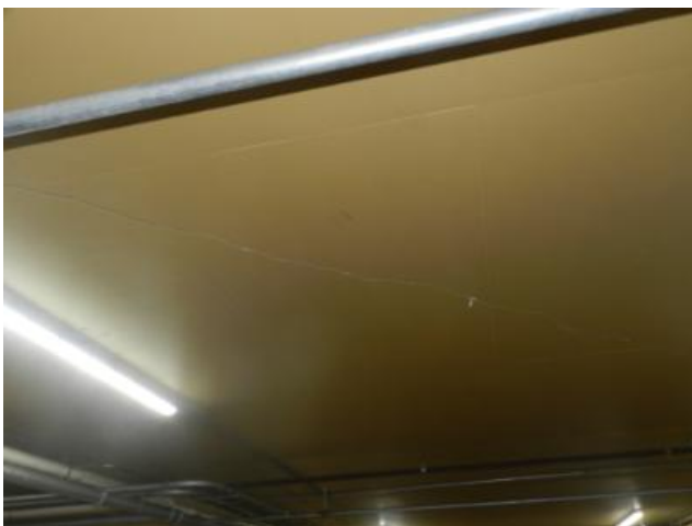
Parking garage ceiling crack.
