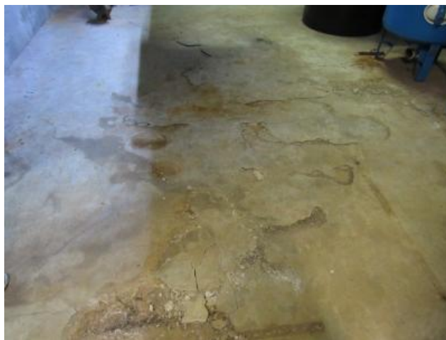
Concrete slab on grade cracks and spalling at the domestic water pump room.
