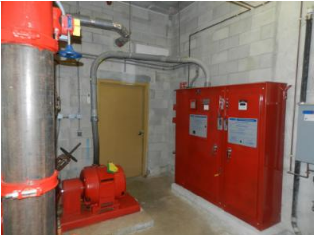
Fire pump main controls.
