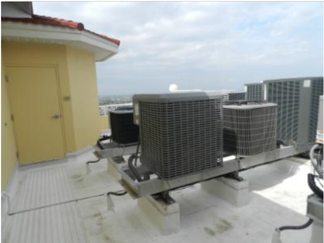
Typical TPO roof covering system, HVAC stands, roof access door, and stone-coated metal panels.
