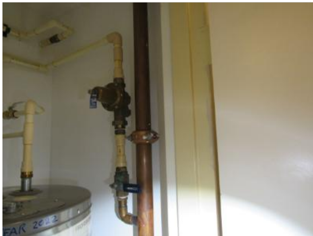
Typical copper and PVC plumbing supply lines.
