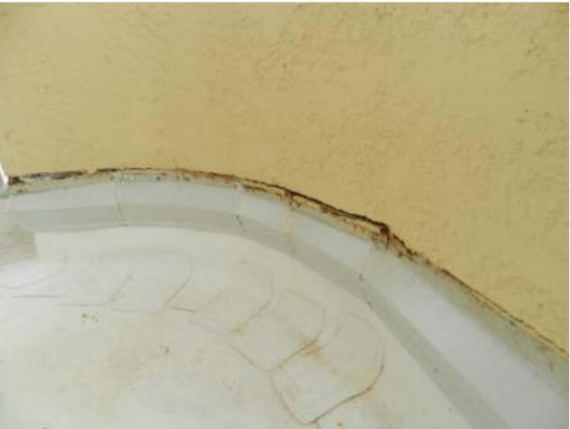
Cracked stucco and rust at the counter flashing.
