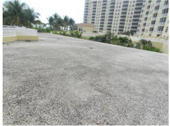
Typical gravel ballast roof.
