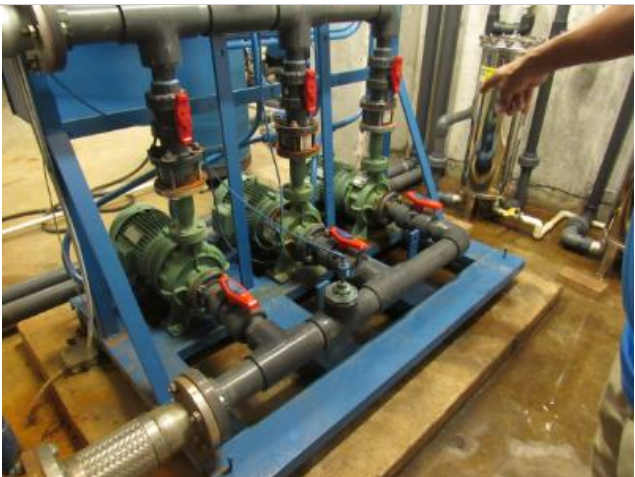
Standing water and apparent leak.
