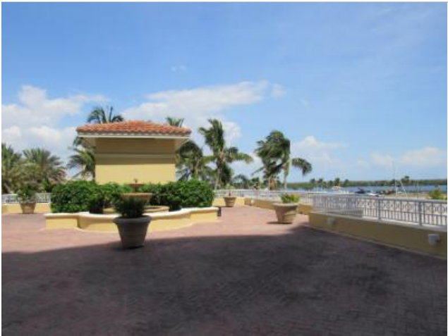
Waterproofed interlocking concrete paver deck and waterproofed planters.
