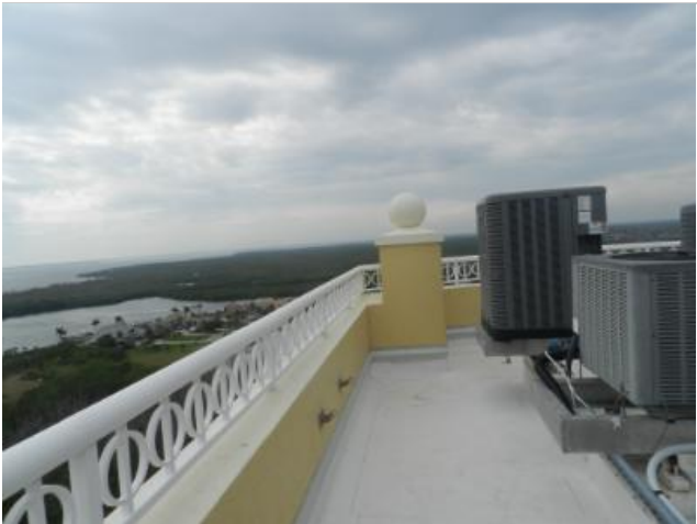
Typical TPO roof covering system, HVAC stands, and fall protection anchors.
