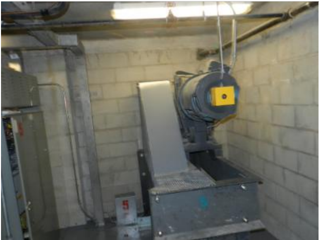
Main traction elevator equipment and controls.
