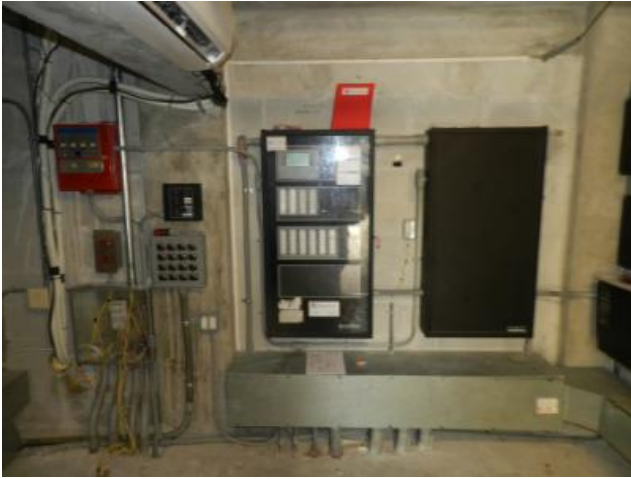
Typical Fire Alarm Control Panel.
