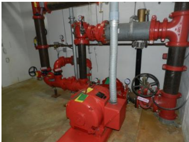
Typical emergency fire pump.
