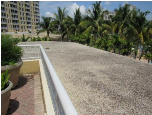
Typical gravel ballast roof and adjacent interlocking concrete paver deck.
