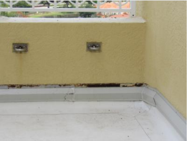
Cracked stucco and staining at the counter flashing.
