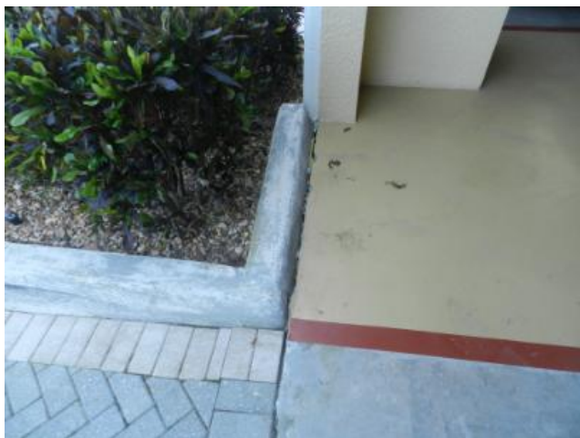
Expansion joint between garage ramp curb and building slab.
