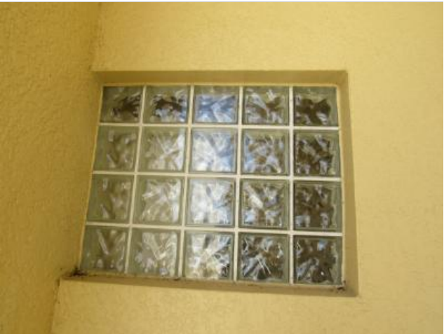
Typical exterior glass block opening.
