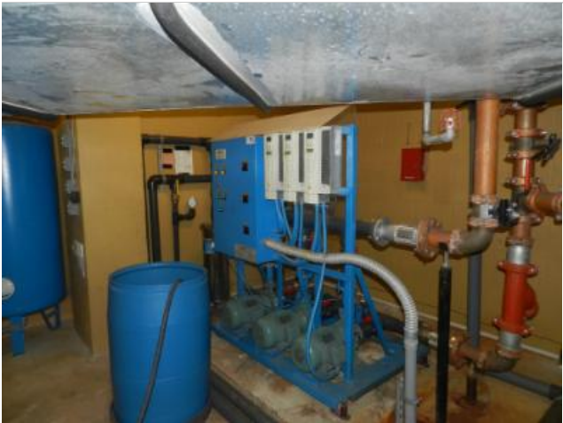
Typical variable speed domestic water pump system.
