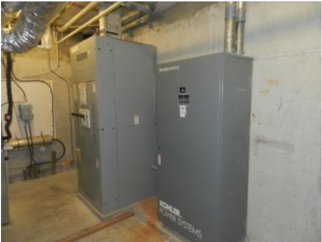
Main electrical disconnects and main distribution panel.
