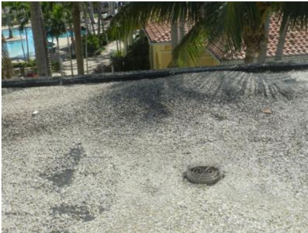
Typical gravel ballast roof. Note area of missing gravel coverage.
