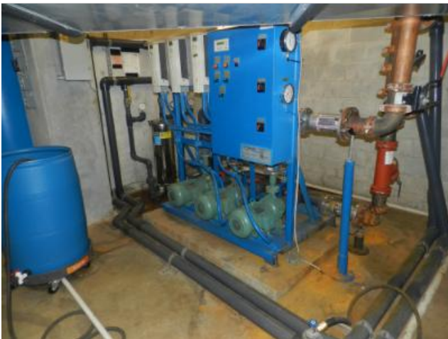
Typical variable speed domestic water pump system.
