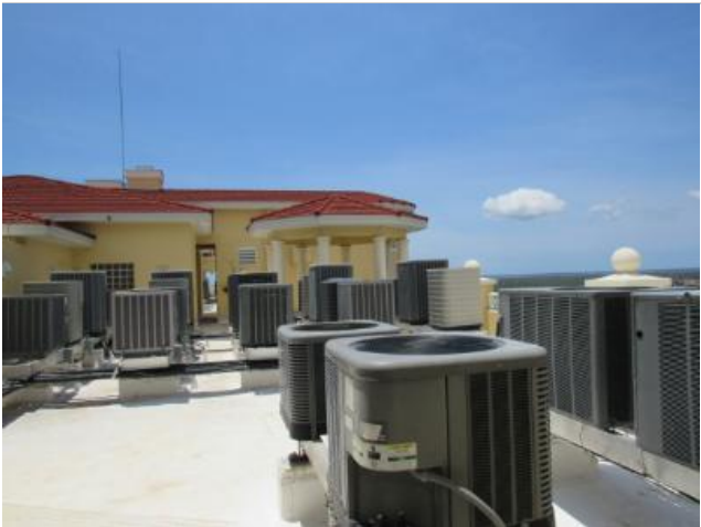
Sloped stone-coated metal panels and flat TPO roof system.
