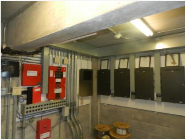
Typical Fire Alarm Control Panel.
