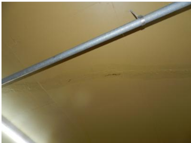
Parking Garage ceiling - Staining and potential signs of water intrusion at a location that was previously repaired.
