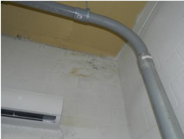
Signs of water intrusion in the fire pump equipment room.
