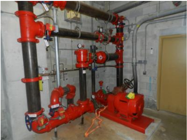
Typical emergency fire pump.
