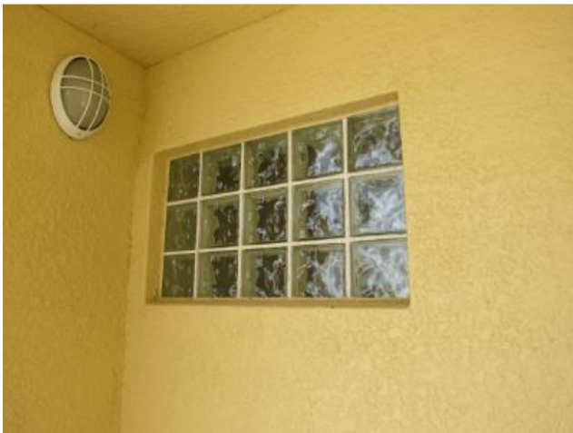
Typical exterior glass block opening.
