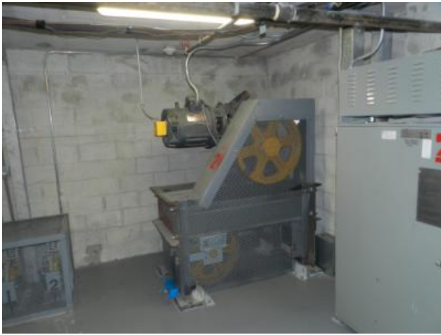
Main traction elevator equipment and controls.
