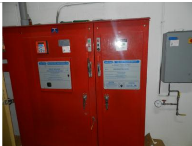
Fire pump main controls.
