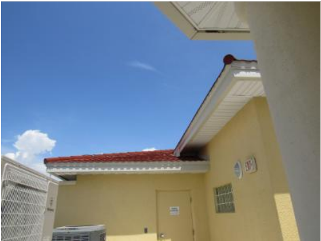
Typical sloped stone-coated metal panels.
