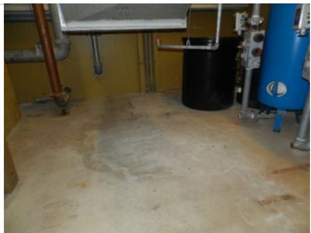
Concrete slab cracks in domestic water pump room.
