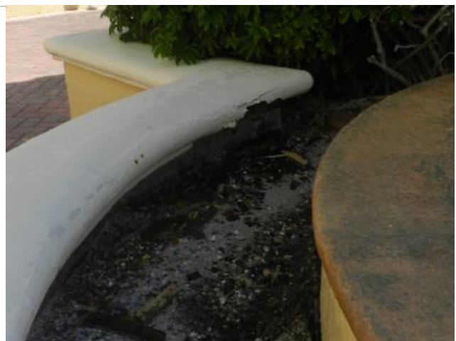
Damaged planter wall cap.
