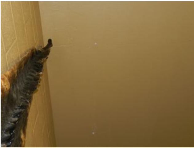
Signs of water intrusion into private garage #56
