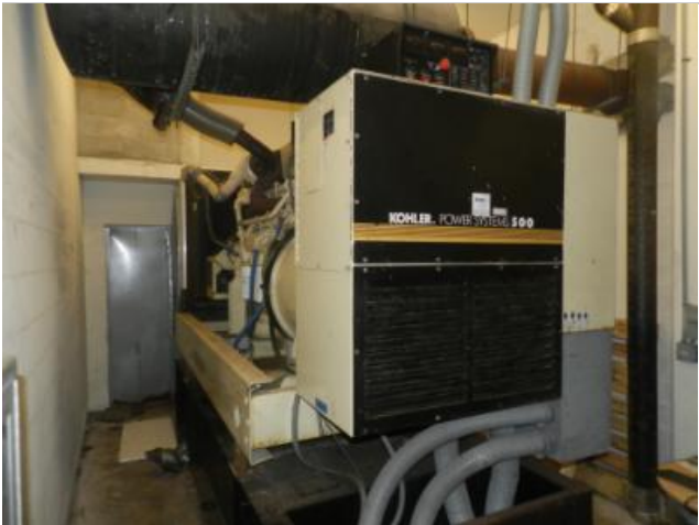
Typical emergency diesel generator.
