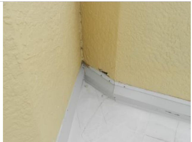
Crack in stucco above counterflashing.
