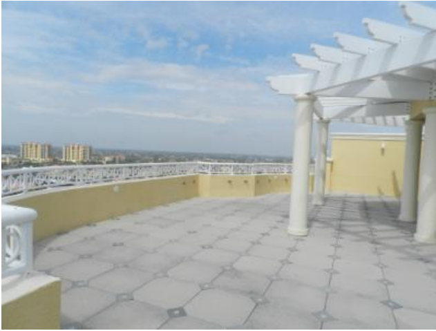
Private Roof Rerrace - Pedestal paver roof system (mod. bit. below pedestal pavers).
