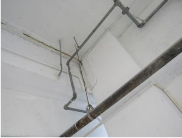
Expansion joint deterioration observed from within the fountain equipment room.
